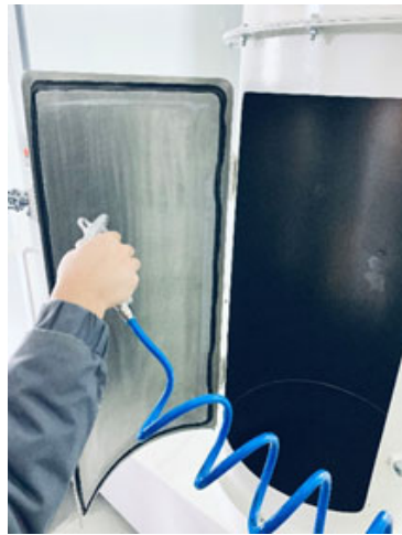
Figure 23 Vertical extract duct inspection door
